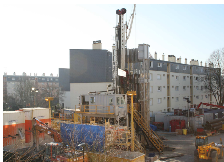
Chantier de forage, Square Fleming
